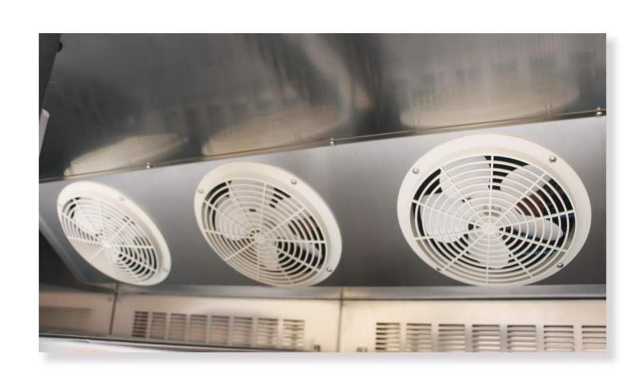
Fan-assisted evaporator and LED lighting
